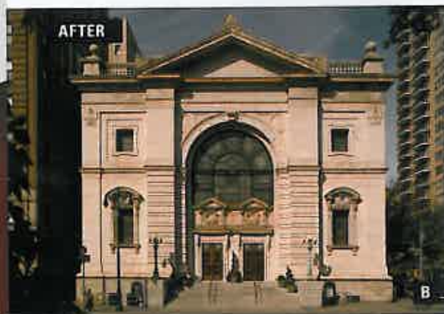
A&B. A before-and-after look at the First Church of Christ, Scientist . Restoration included cleaning and repointing the façade, which consisted of a Concord White granite base and water table, as well as Dover White marble façades. Photos courtesy of Sydness Architects
